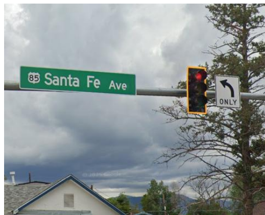
Retroreflective Backplate for the traffic signal at Santa Fe Avenue and Indiana Avenue
